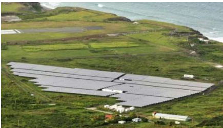
Example 1: Island electrification (St. Eustatius) with 4.1 MWp PV plus 6 MWh Li-ion battery storage
