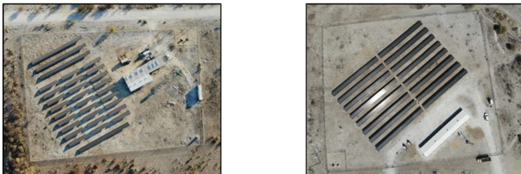
Figure 1: PROCEED's reference objects in Tsumkwe (left) and Gam (right) in the Otjozondjupa region in northeast Namibia are currently the country's largest mini-grid systems (images: Fabian Junker, THI)
